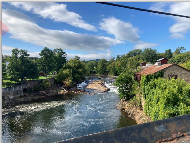
Ausable River, captured from the Stone Arch Bridge
